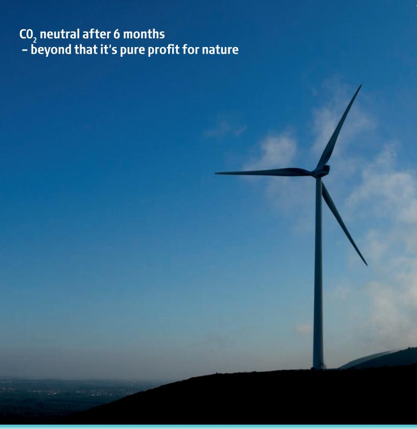
After 6-9 months a Vestas V90-3.0 MW wind turbine has produced the same amount of energy as it uses in its entire lifetime.
